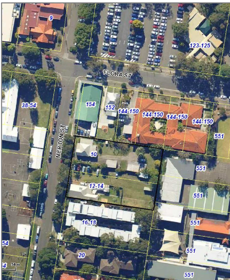
Figure 1: Aerial view of the subject site
